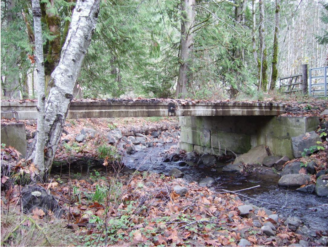
Picture 1: Upstream of the bridge, looking downstream.
