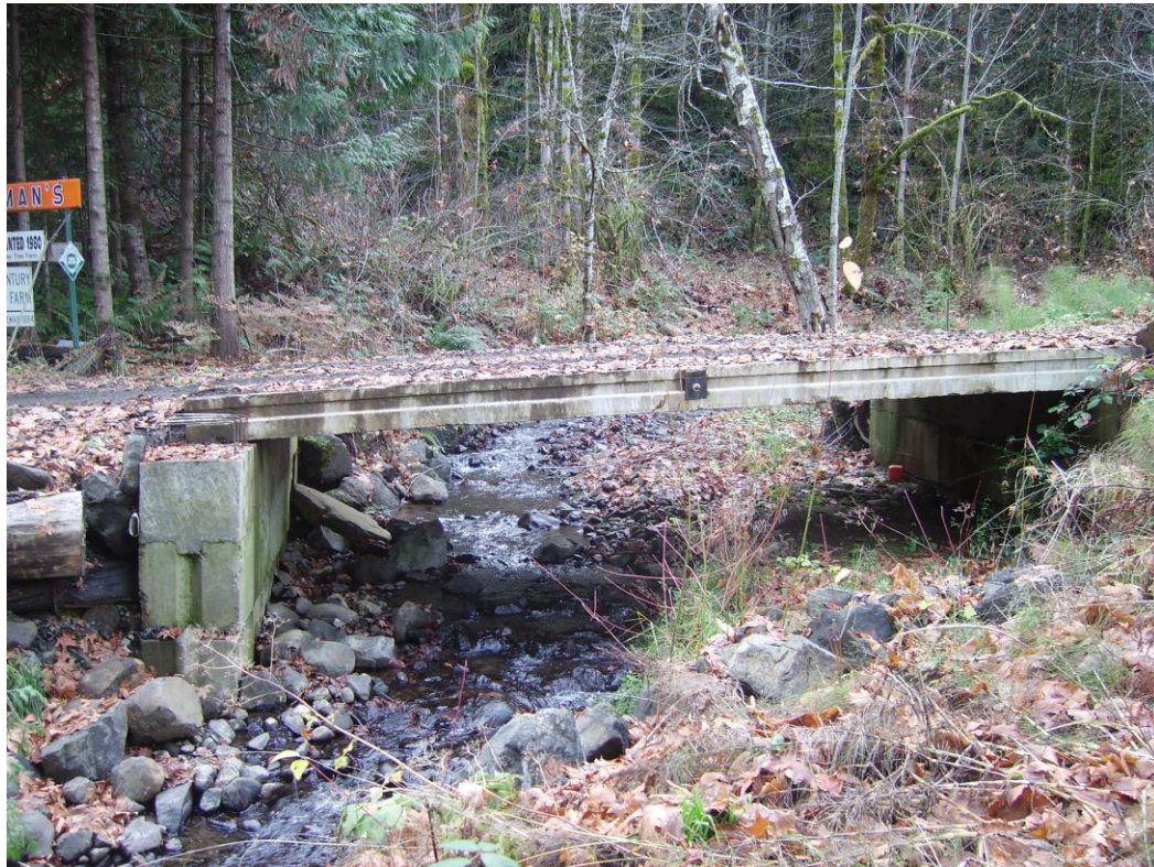
Picture 2: Downstream of the bridge, looking upstream
