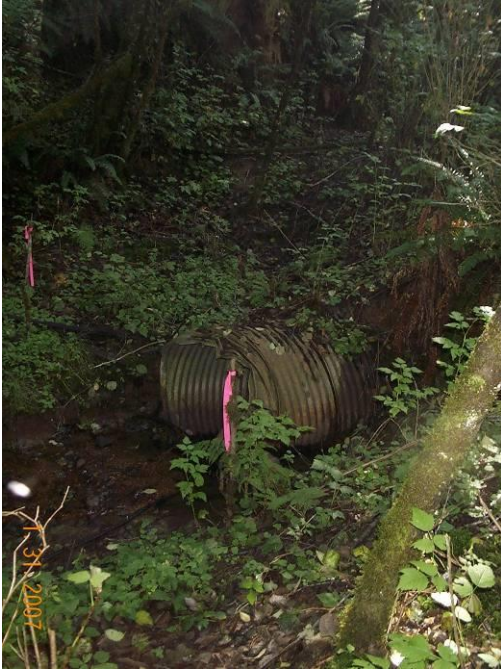
(Pre-Project): Most upstream end of West Fork Dairy Creek culvert.
