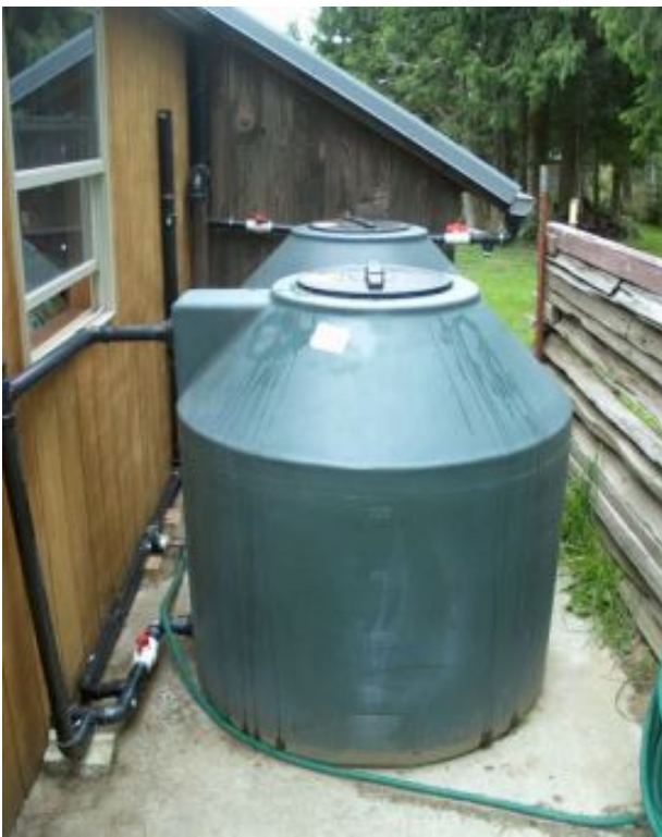
Large (>550 gallons) rainwater harvesting system pictured above, and small (55 gallons) rain barrel systems pictured to the right.
