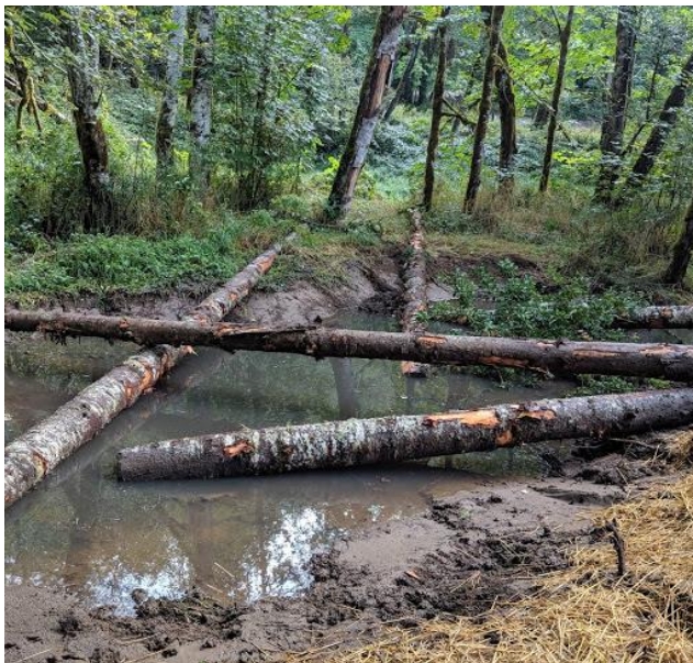
Figure 1. Large wood in excavated alcove.
