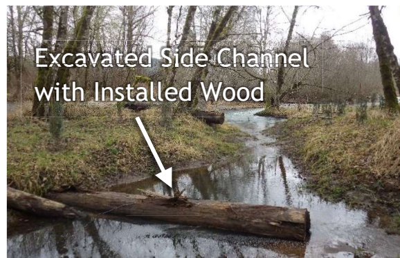
Views of the notched dike (top) and excavated side channels with installed large woody materials (bottom) constructed in summer 2018 (photos by Stillwater Sciences)
