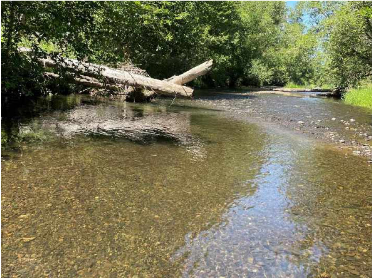
Photo 4: Gales Creek mainstem treatment logs functioning as scour vectors
