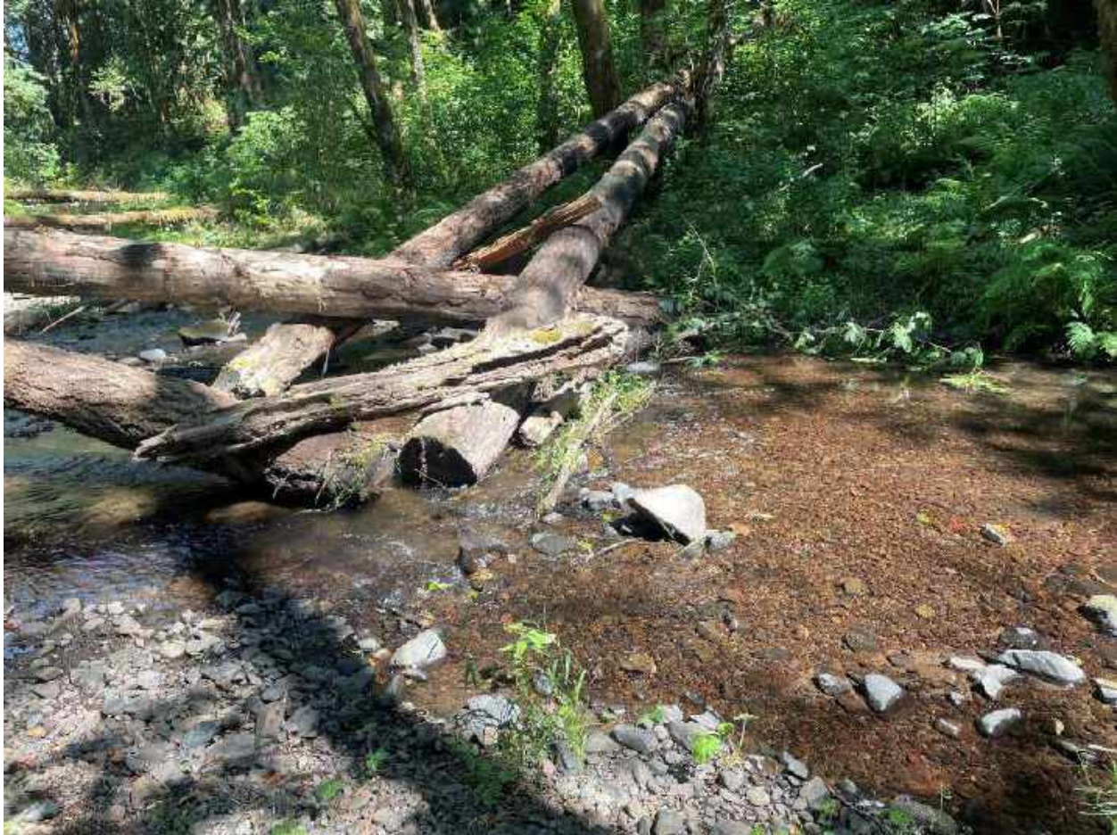
Photo 13: Clear Creek, 2021 LWD treatment with gravel accumulation
