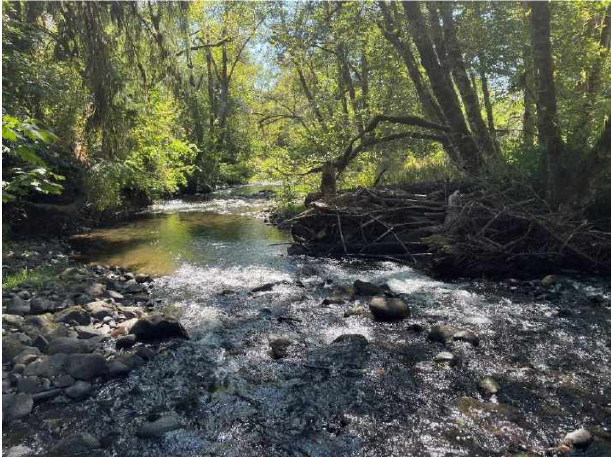
Photo 24: East Fork Dairy treatment logs collecting debris and functioning as scour vectors
